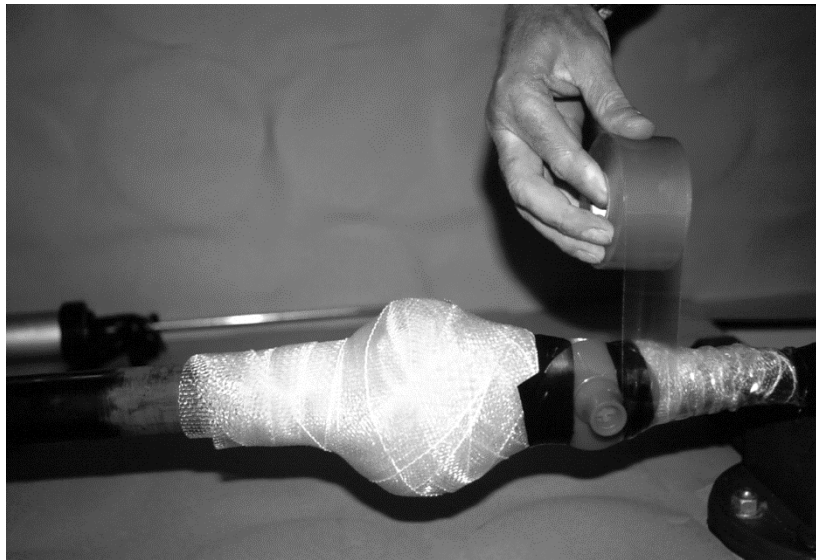
Mounting of cable joint.
